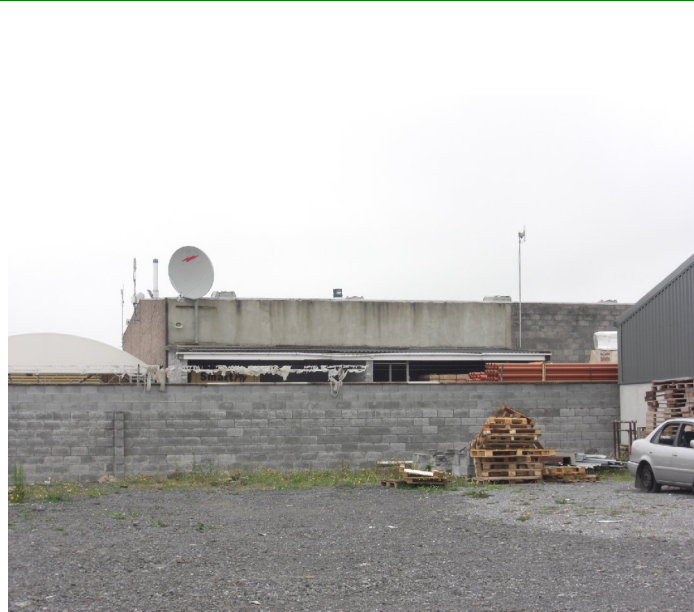
Transmitter Site Photo
